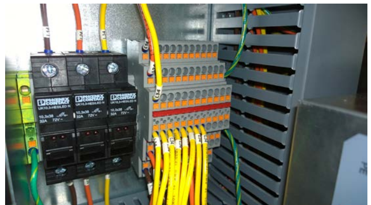
Figure 3: The 3-mm terminals have three levels, which "makes three-phase wiring a breeze," according to Forpak. To release the connections, the user simply presses on the orange actuation lever.
